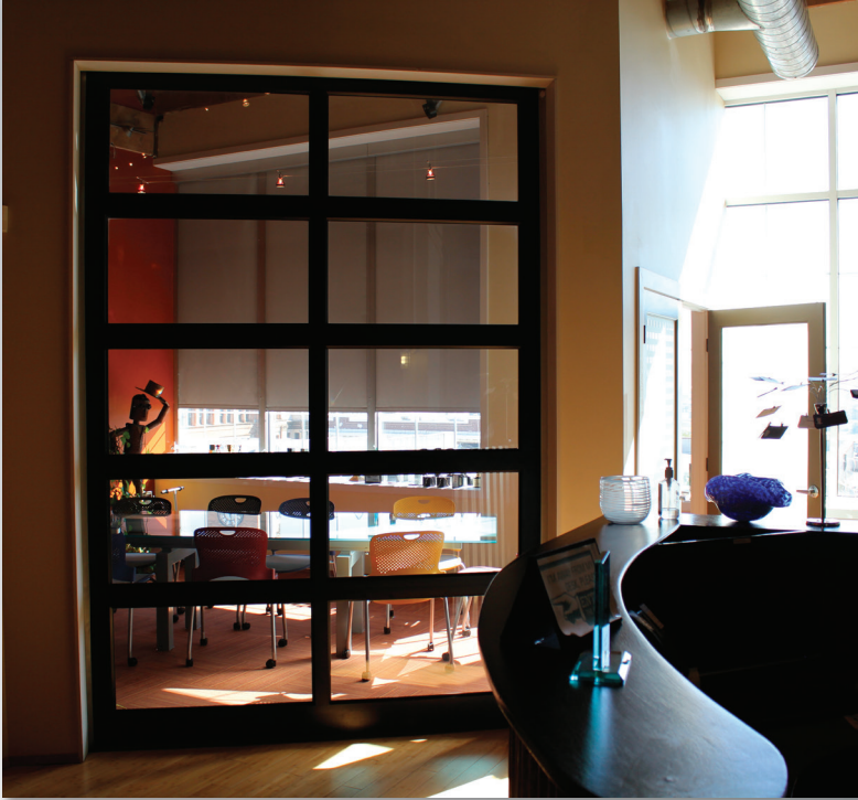
Model MC52-SC used to separate a conference room from the reception area. It has a Black Anodized finish and Clear Tempered Glass panels. This door has been in use for over seven years and still looks brand new.
